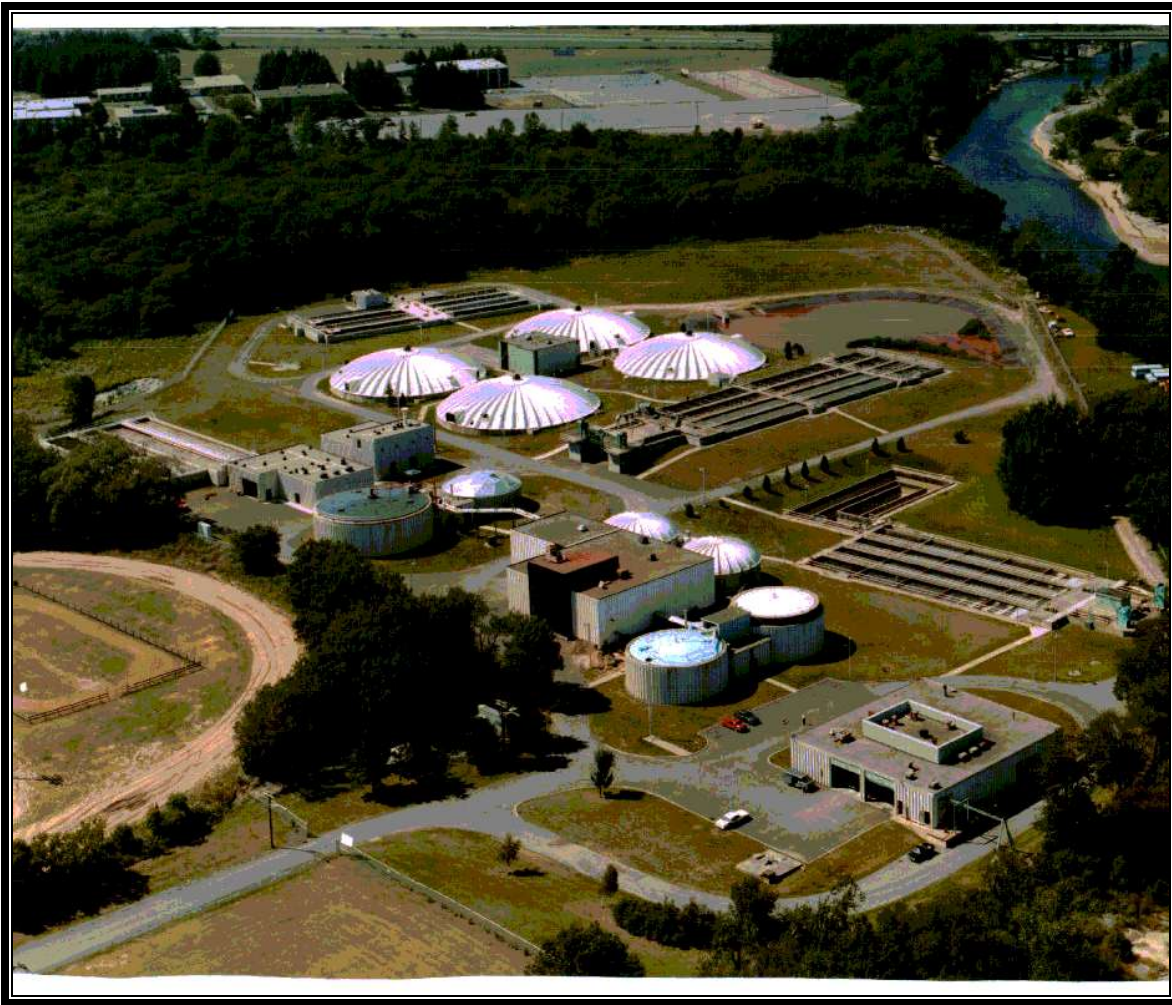
Figure 4: Aerial of the Watertown Pollution Control Plant
